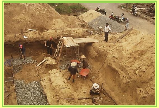
The workers constructed the wooden frame molds and filled them with gravel and layers of cement.
