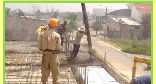
The front canopy would be too heavy if it was filled with solid concrete only. Blocks of foam were used to make it lighter.
