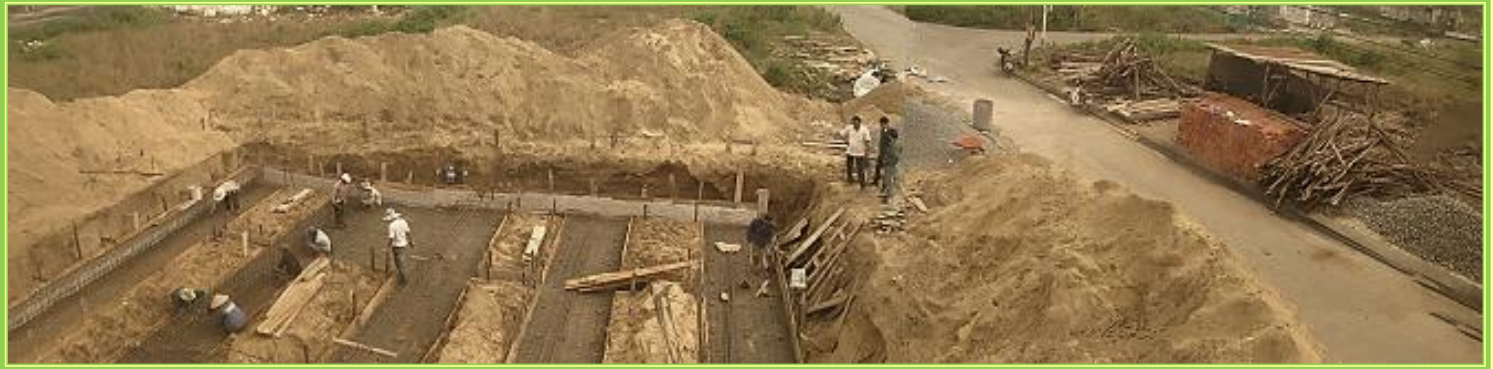
The next step was filling the molds with concrete iron bars
