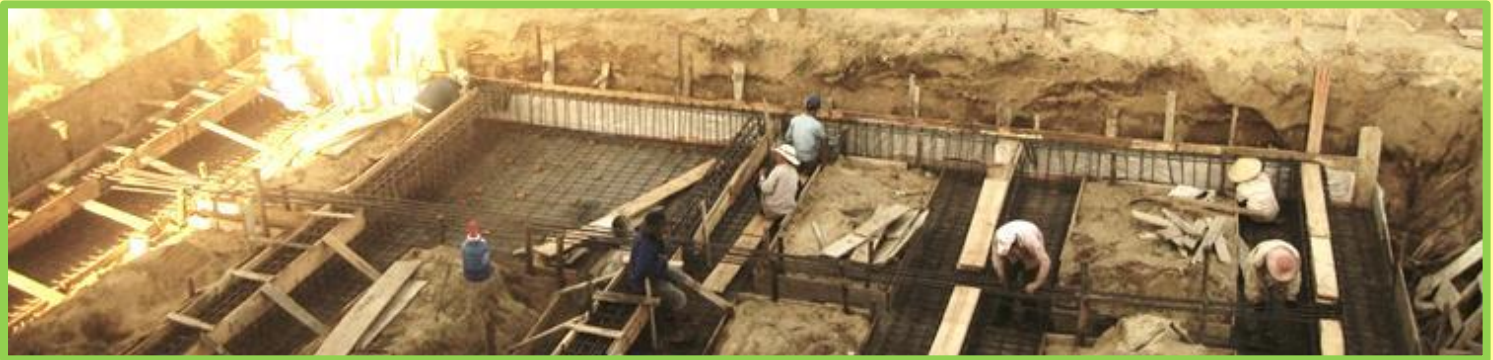
Hard work but very rewarding. Making the foundation ready to be filled with concrete cement.
