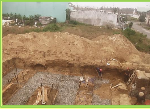
The workers constructed the wooden frame molds and filled them with gravel and layers of cement.
