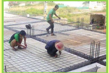
Tons of iron has been used for the ceiling. It took a while before it was ready to be filled with concrete.
