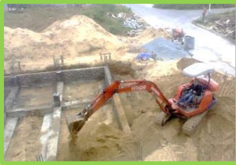
The foundation was filled up with sand, making it ready for the 24 pillars to be constructed
