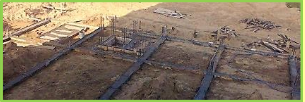
The foundation was filled up with sand, making it ready for the 24 pillars to be constructed
