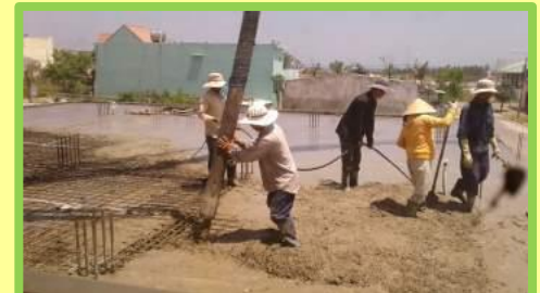
Again we hired a truck with a concrete pump to fill the ceiling frame molds.
