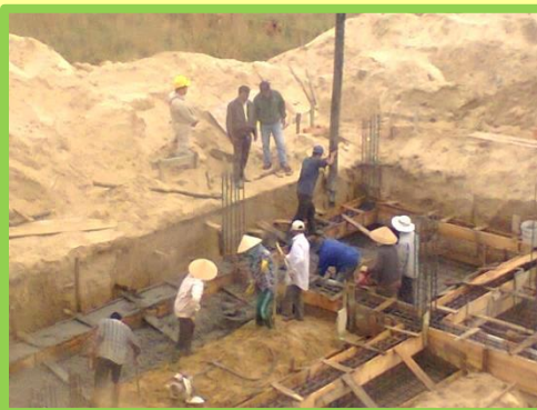
Nine beton mixer trucks were needed to fill the frame molds with the help of a modern concrete pump.
