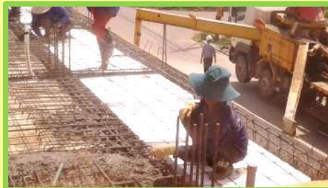
The front canopy would be too heavy if it was filled with solid concrete only. Blocks of foam were used to make it lighter.
