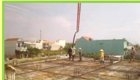
Again we hired a truck with a concrete pump to fill the ceiling frame molds.
