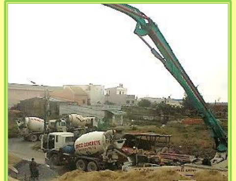
Nine beton mixer trucks were needed to fill the frame molds with the help of a modern concrete pump.
