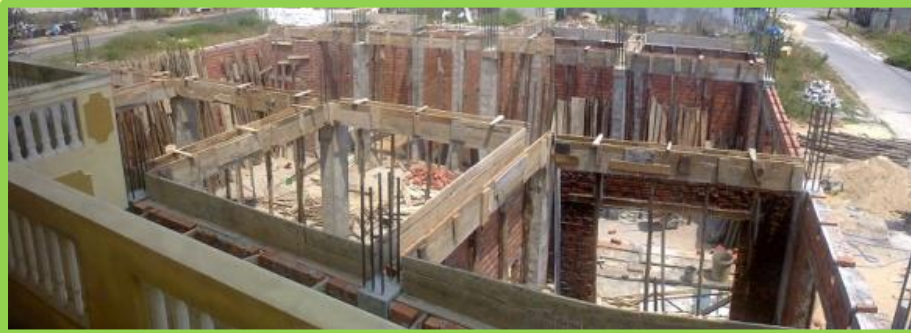
After one month the wooden molds of the ceiling were built.
