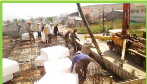
The front canopy would be too heavy if it was filled with solid concrete only. Blocks of foam were used to make it lighter.
