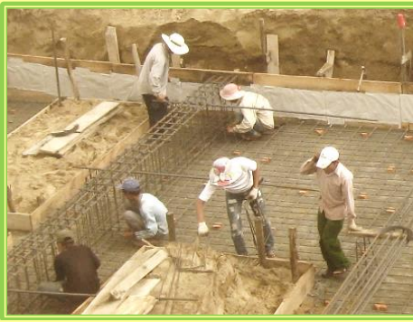
The workers constructed the wooden frame molds and filled them with gravel and layers of cement.
