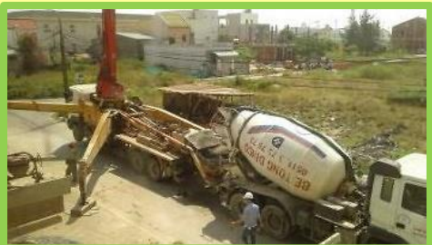
Again we hired a truck with a concrete pump to fill the ceiling frame molds.
